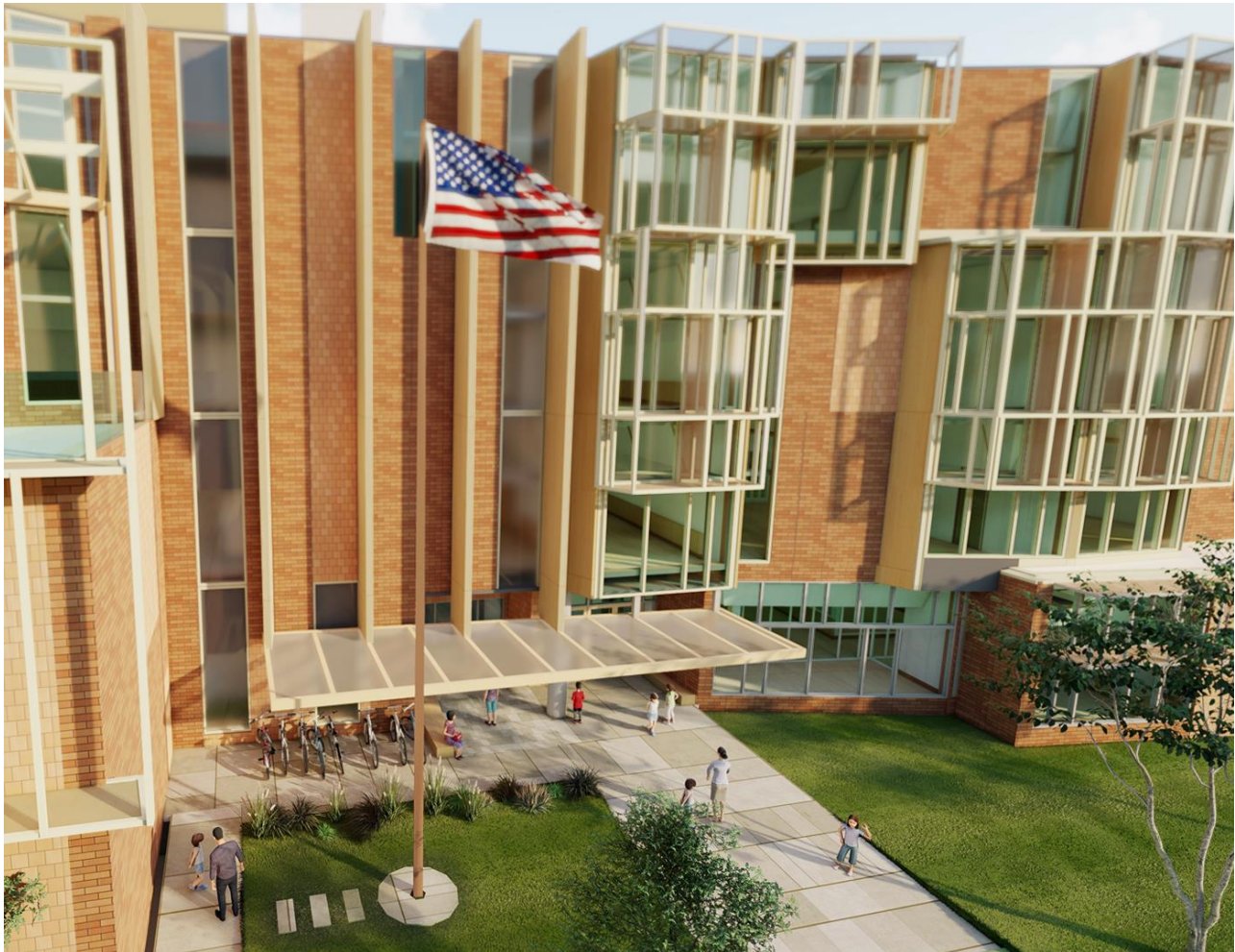
Washington Street Entrance
